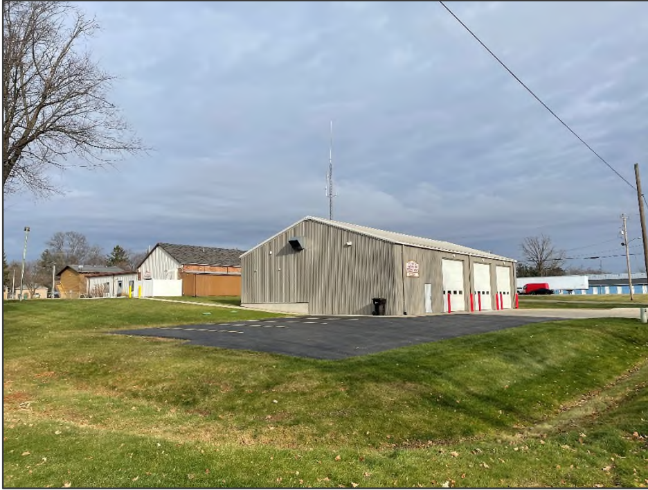
PHOTO NO. 31: View of the fire department at 16-403-009-00 (13551 15 Mile Road).
