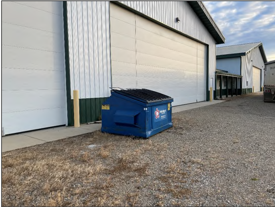
PHOTO NO. 17: View of the general waste dumpster located south of the structure at 16-281-021-00 (14219 C Drive North).
