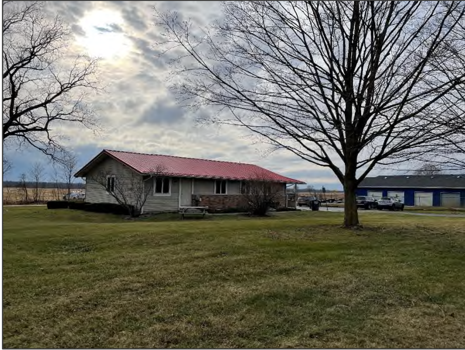
PHOTO NO. 1: General view of the Subject Property from the northeast corner.
