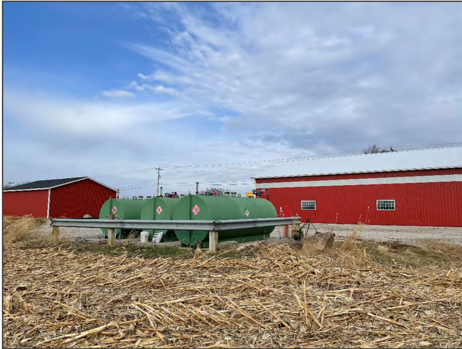
PHOTO NO. 29: View of the agricultural structures and three 3,000-gallon diesel fuel ASTs at 16-281-015-05.
