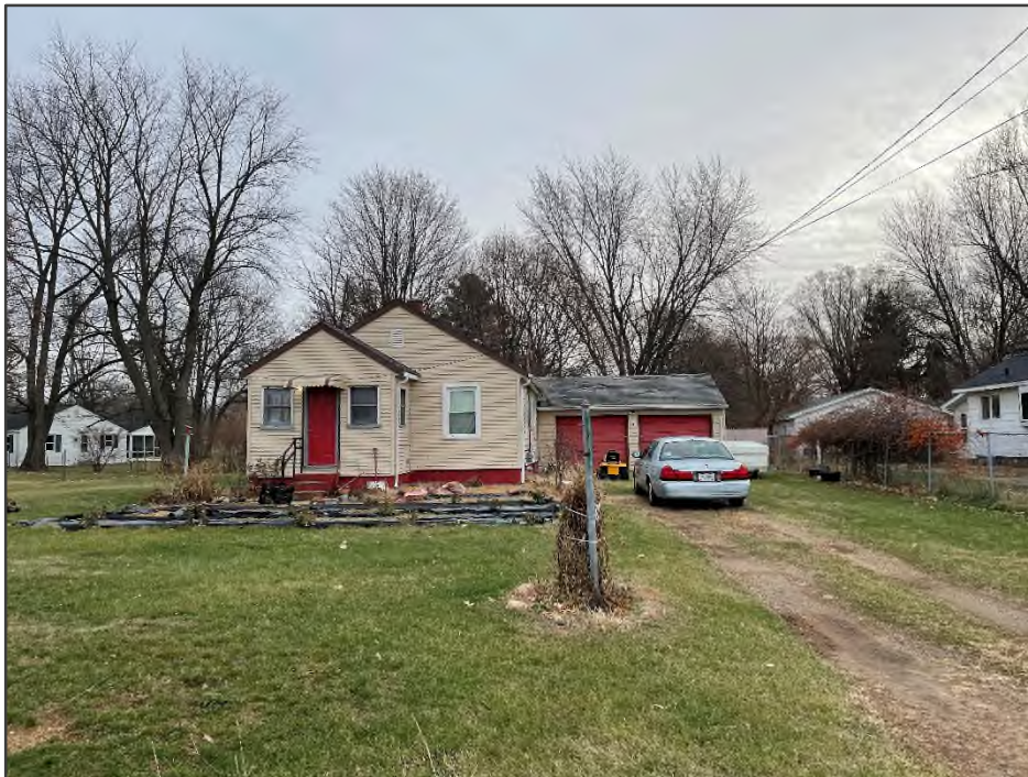
PHOTO NO. 10: View of a typical residential structure.
