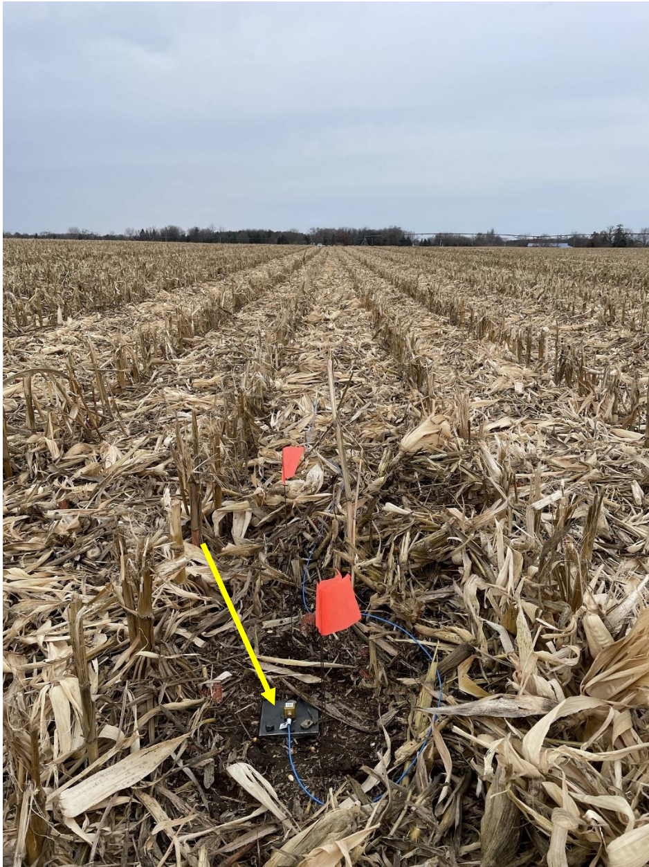
Figure 7. Typical accelerometer (yellow arrow) installation with marker flags.
